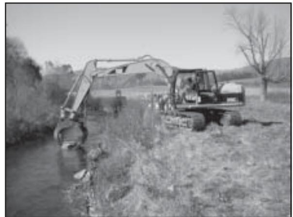
*Downstream area during construction of rock vein.*
