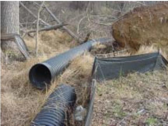
*An uprooted tree was the cause of this slope pipe being disconnected.*
