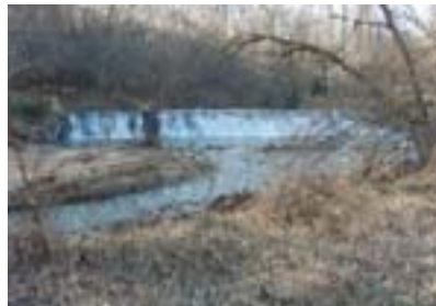
Irving Mill Dam in January 2004
