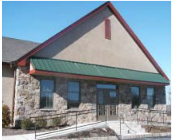
The newly constructed offices of the Bucks County Conservation District in Fountainville.
