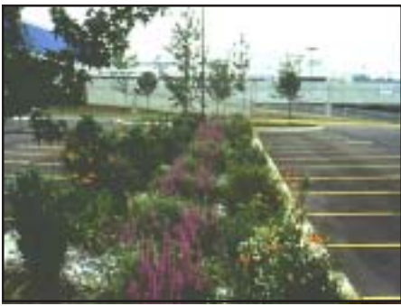
Bioretention landscaping reduces water runoff and beautifies parking areas.
