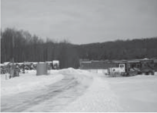
Containment tanks for frac water at a well pad site in Susquehanna County
