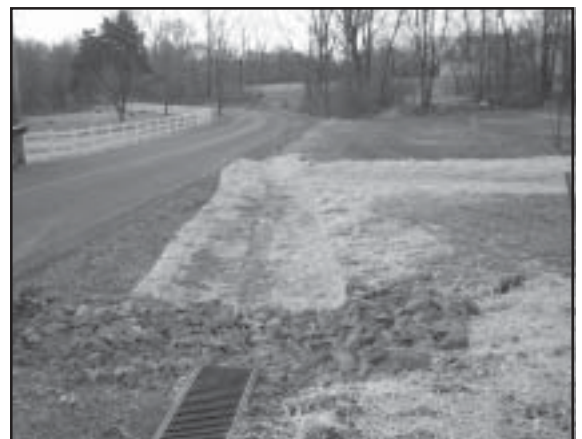
Install lining for better erosion control.
