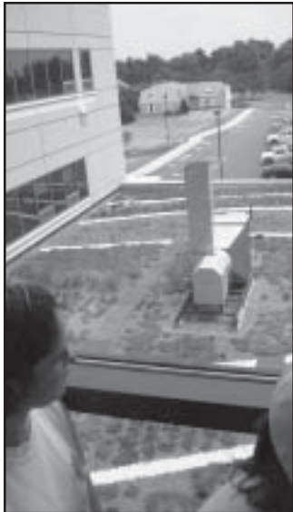
Bonnie Tobin of Delaware Canal State Park looks down on the green roof at St. Mary's Hospital in Langhorne
